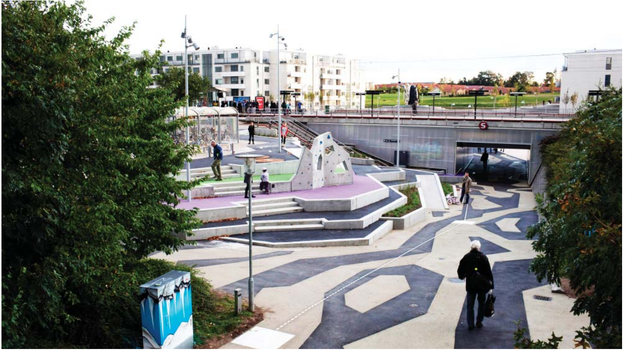
Image caption: ADEPT/LiWplanning, Måløv Axis, By the Måløv Station a huge leap of a stair/ramp construction encouraging recreational and social activities
